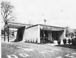
Quincy Motor Bank 60 McGrath Highway
